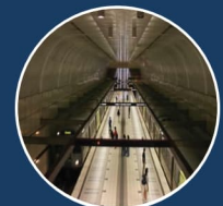
Tren Urbano Underground Station (Rio Piedras) San Juan, PR
