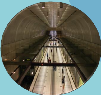
TREN URBANO UNDERGROUND STATIONS RIO PIEDRAS SAN JUAN, PR
