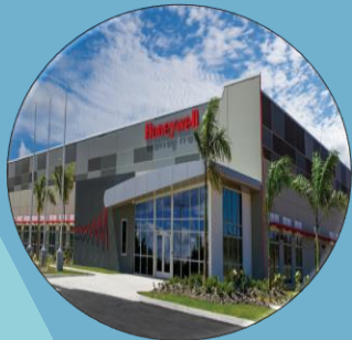
HONEYWELL AEROSPACE ENVIRONMENTAL TESTING LAB MOCA, PR
