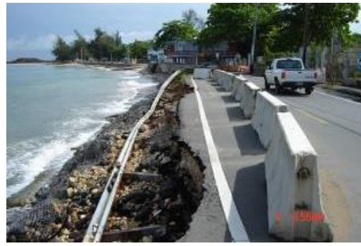
Erosion Conditions threatening the structural integrity of the road and jeopardizing the community's safety.
