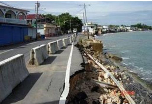
Erosion Conditions threatening the structural integrity of the road and jeopardizing the community's safety.
